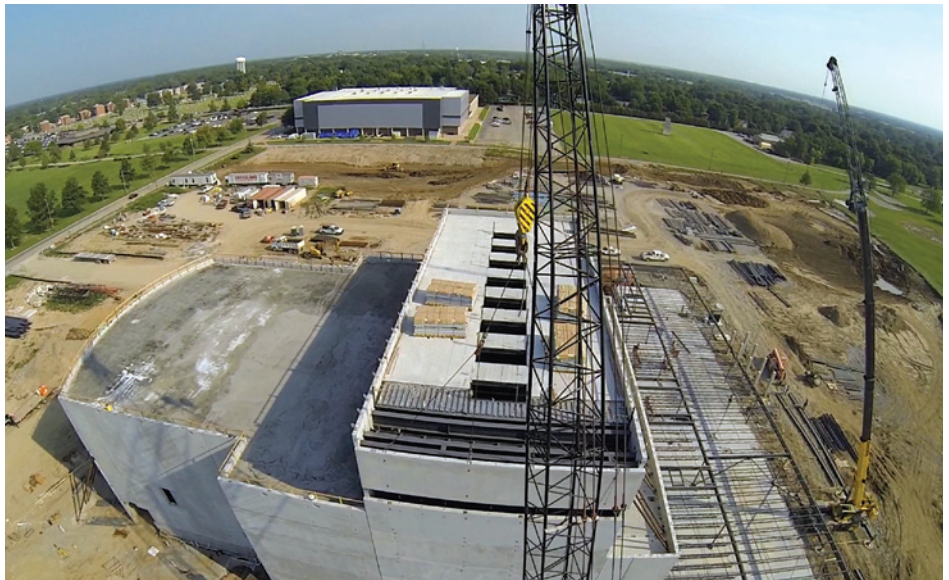
Cranes lift steel and pre-cast concrete panels more than 70 feet into the air for installation on the Center for the Arts. This view looks north, with the Weede PE Building in the background.
